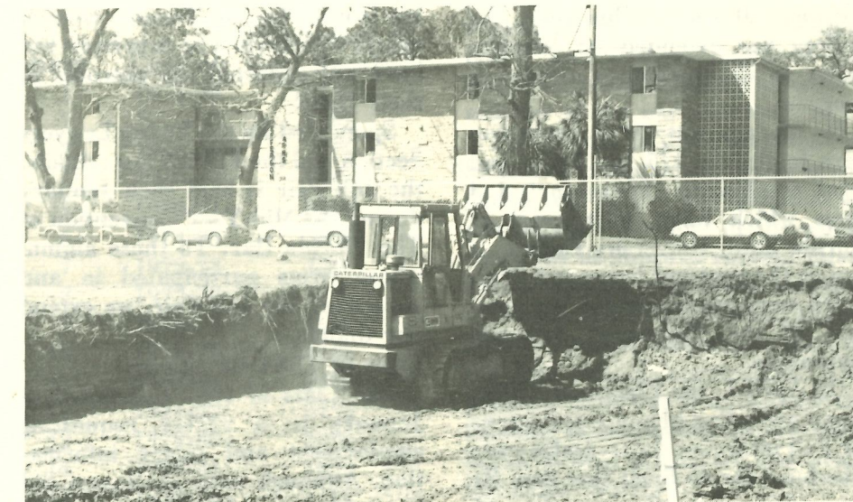
Excavation site for first house in Village Green.
