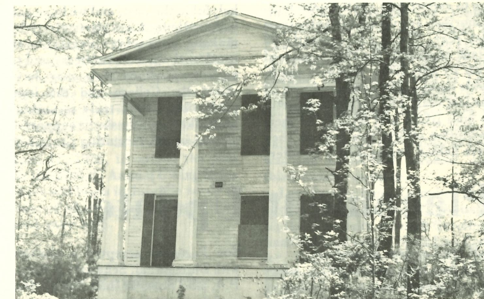
View of Hobby-Harrison House before being moved to law school campus.
